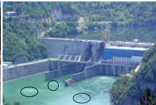
Fig. 5: Boils in the river bed downstream of the dam
