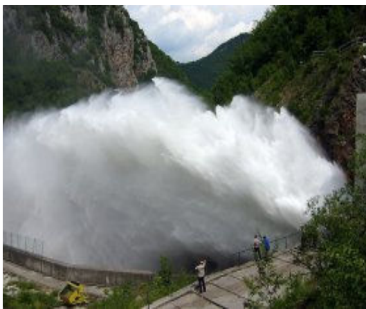
Fig.6: Low level outlet in operation
