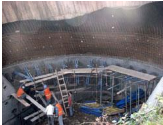
Fig. 9: Repairs of the arches
