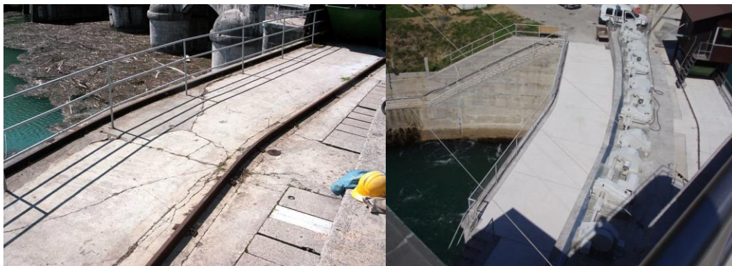
Figure 6 pavement of the intake structure before rehabilitation in 2004 and after it
