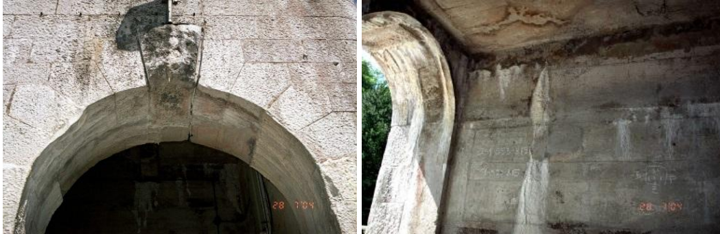
Figure 4 Stone facing with joints filled with flowstone in 2004
